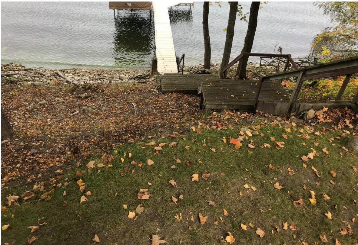
Steep eroded hillside. Project will stabilize using native seed and erosion blanket.
